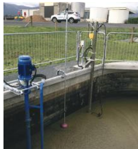
Submersible Stirrer and Lifting frame on Sump application.
