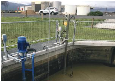
Submersible Stirrer and Lifting frame on Sump application.
