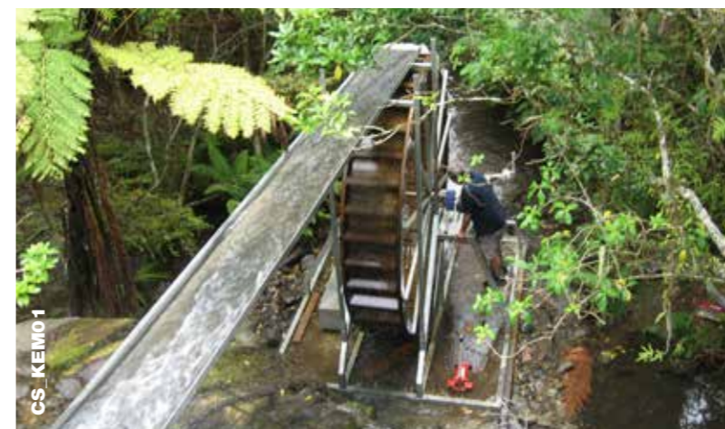
15' x 2' Yardmaster Water Wheel featured construction using Kauri timber supplied by client. (see cover image)
